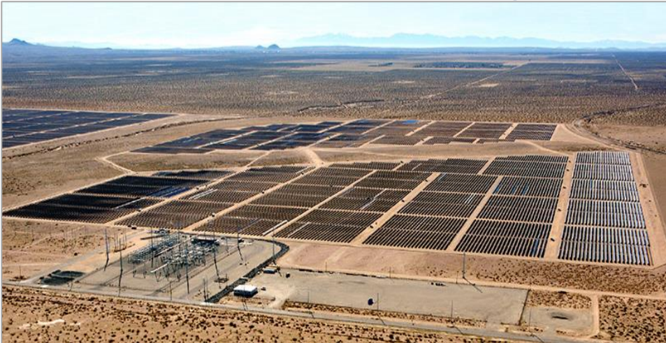
* Beacon Solar Plant, Mojave, California US.
