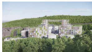
Bundang CCPP (Modernization)
