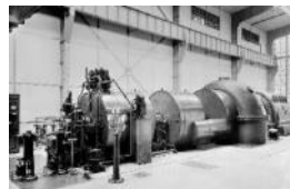
The first Doosan 412kW steam turbine; System Rateau
