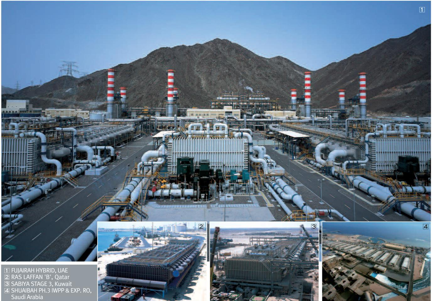
Accounting for approximately 80% of the solutions provided by the seawater desalination industry, Multi-Stage Flash (MSF) has been playing a major role in providing fresh water resources in the Middle East. The MSF process generates potable water from seawater using a flashing method, which creates instantaneous discharging of water vapor.
