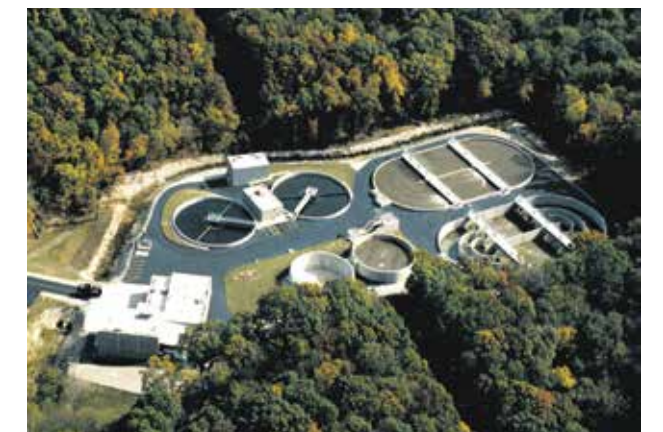
Water Treatment System
