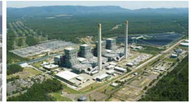
Eraring Power Station in Australia
