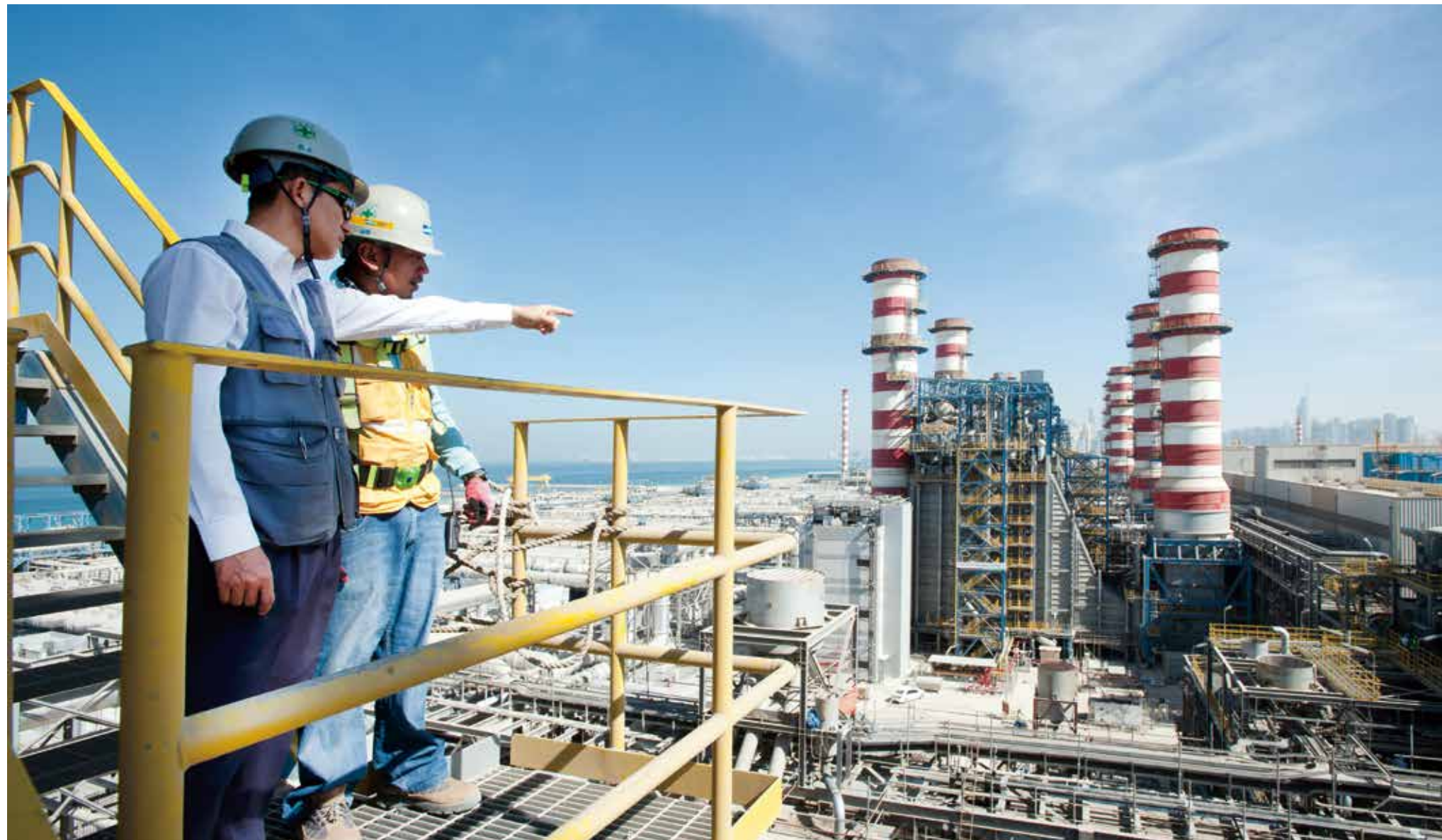
UAW, Jebel Ali M Combined Thermal Power Plant
