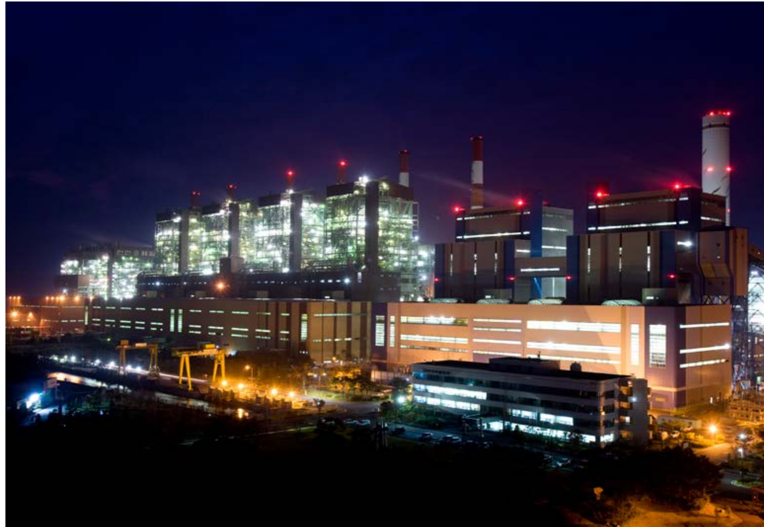
Boryeong Thermal Power Plant Units 3 &amp; 4
