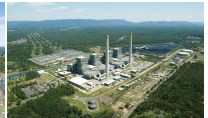
Eraring Power Station in Australia
