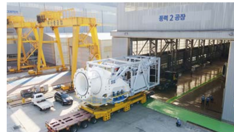
Wind Turbine Shop #2 at Changwon Headquarters
