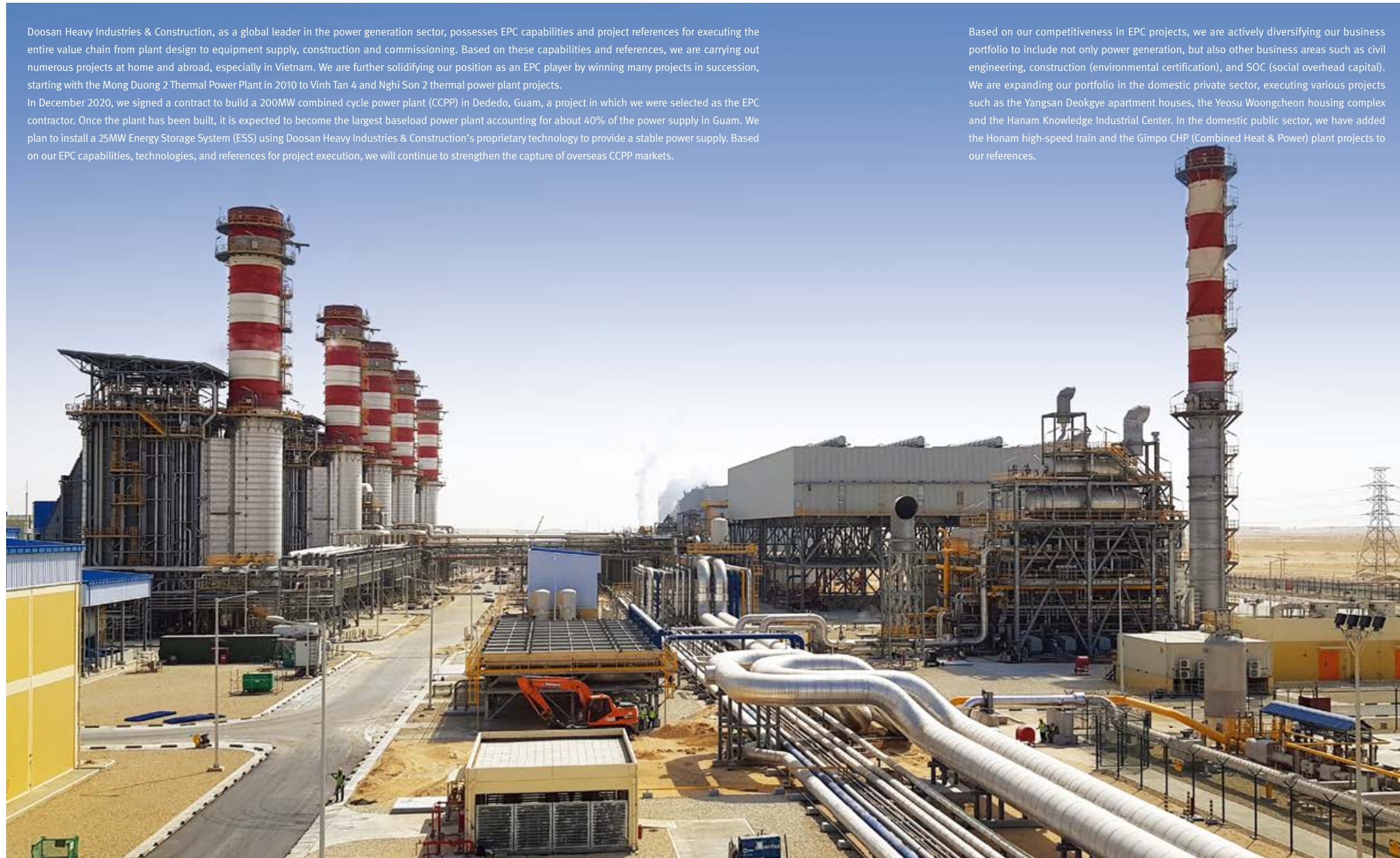
Fadhili Combined Cycle Power Plant in Saudi Arabia
