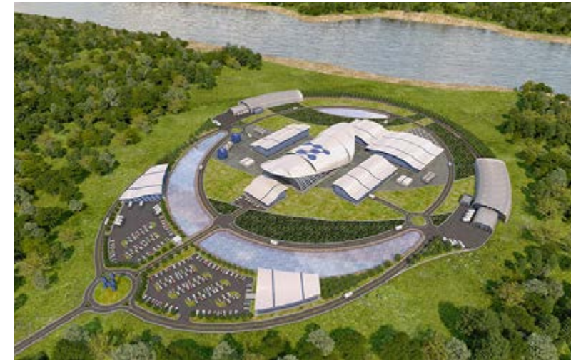
Aerial View of NuScale SMR Plant
