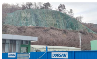
Rockfall-Prevention Structures on Rock-Cut Slopes
